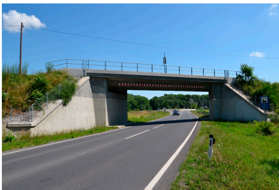
Figure 2. Case study—the Weikendorf Bridge, side view after the repair in 2014.
